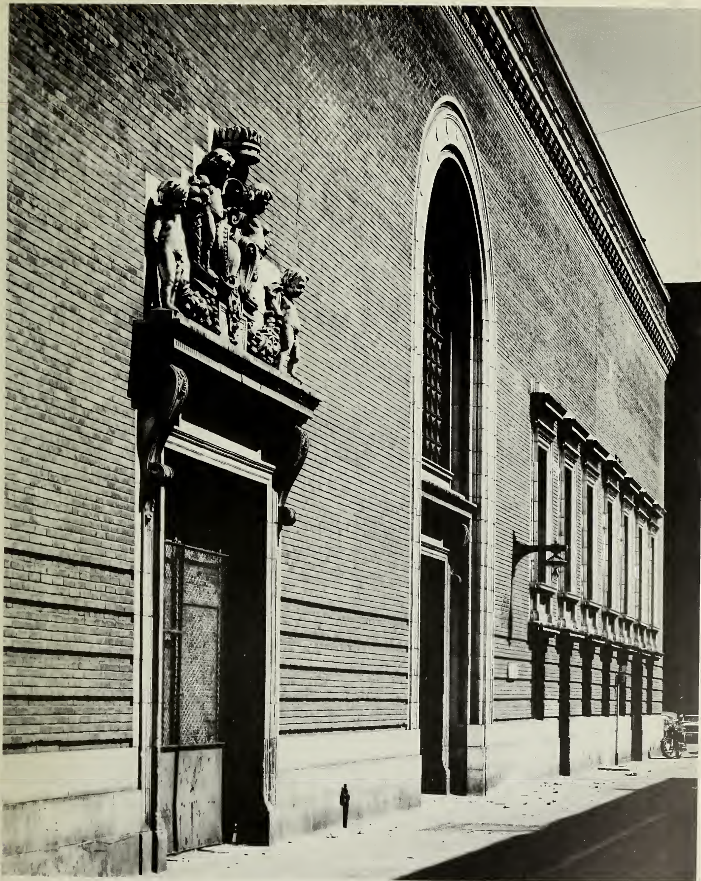
Plate 72: The Jessie Street Substation . . . Designed by Willis Polk and erected by P.G. & E. in 1907, this hidden architectural jewel of the city is now splendidly visible from Mission Street. (Morley Baer)
